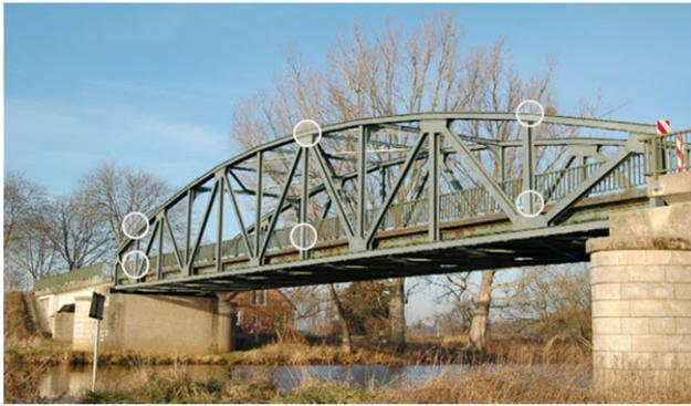
Fig. 3: Typical truss bridge with marked hot-spots
